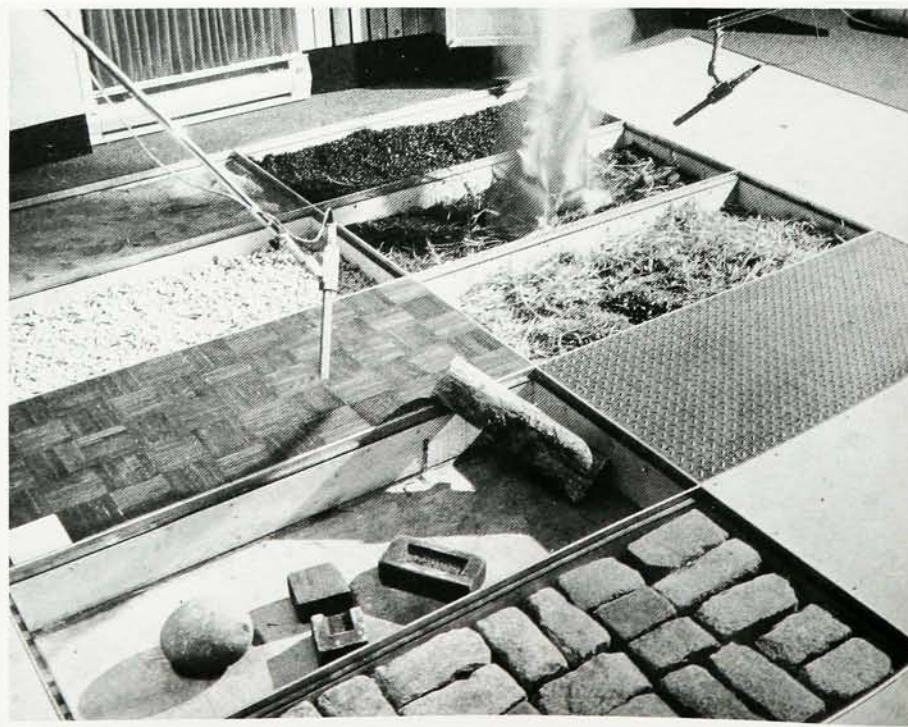
Multiple floor surfaces under the carpet in Studio B, to replace the movement sounds.
