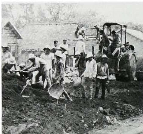
A road-building crew
